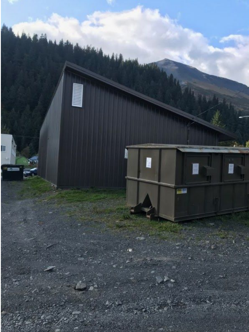
Recycling container and the NPS building it sits next to.
